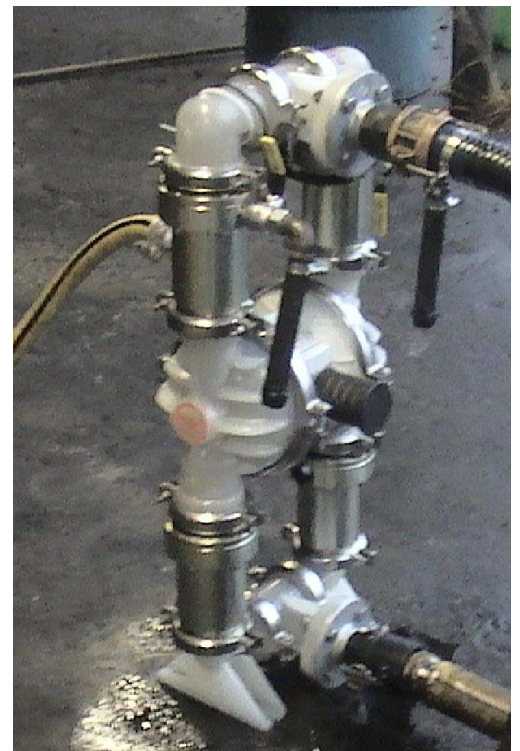
The new valves shown installed on a standard diaphragm pump
